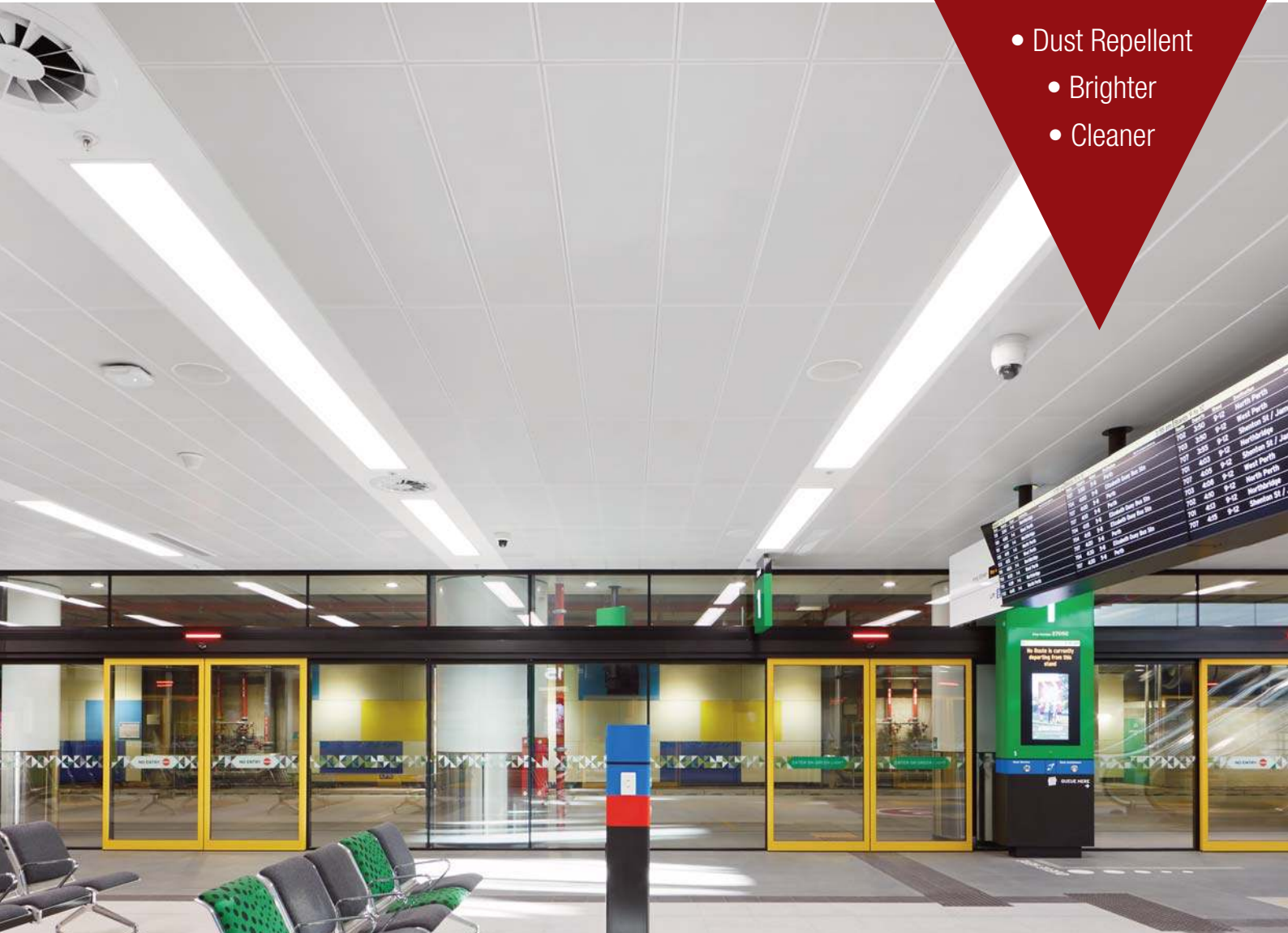
Image: METALWORKS Clip In Ceiling installed at Perth Bus Terminal, WA
