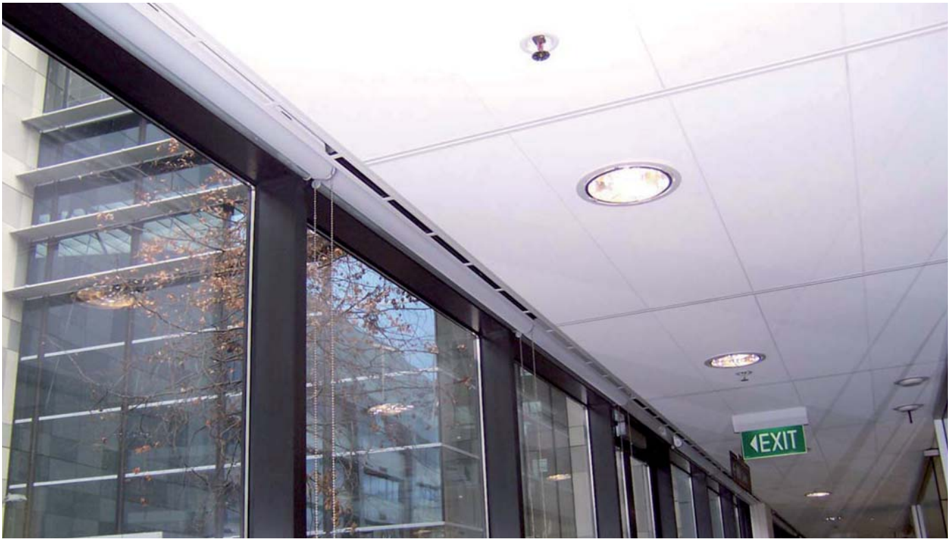
3-Sided Pelmet with slotted Air Diffuser Face Plate – Modular Grid and Ultima panel – Woolworths HQ, Sydney
