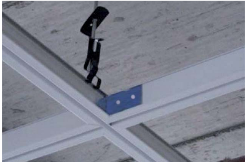
Clean mitred cross runner intersection.
